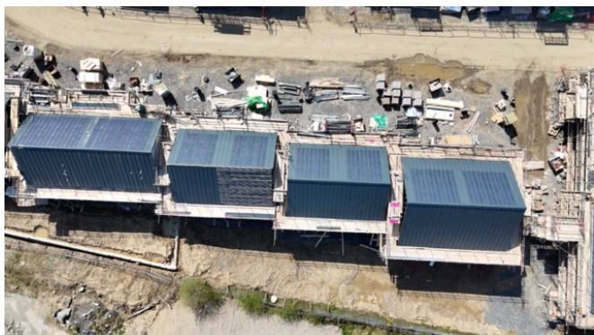
The steel-framed homes we’re building at Pemberton feature Catnic Solarseam roofs that provide the benefits of solar panels whilst meeting the highest fire safety requirements.
